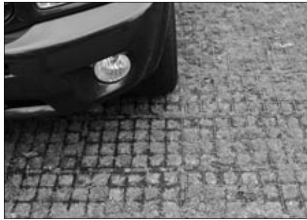
Permeable paving made of recycled plastic enables rain water to soak into the ground naturally, rather than into the municipal drain system.
