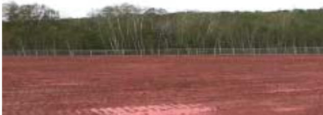
Mason Sands currently undergoing remediation.
